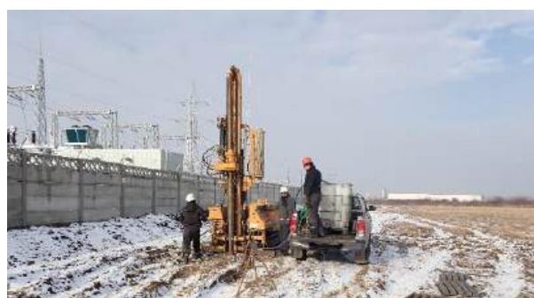
Fig. 8. Execution of borehole FS02
